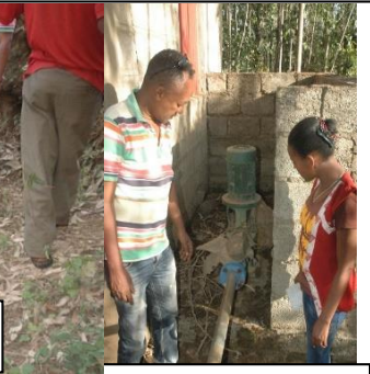
Pump might be working but no water to the wet well to pump
