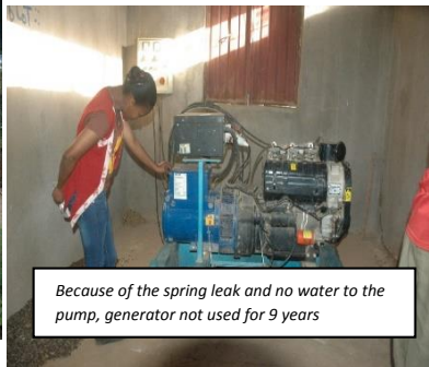
Pump might be working but no water to the wet well to pump
